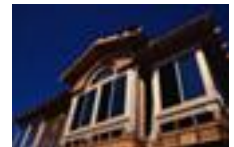
House Under Construction HIM0028
