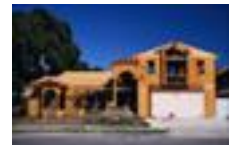
House Under Construction HIM0029
