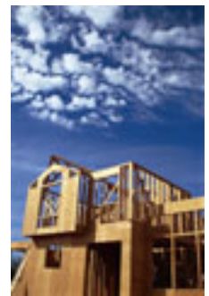
House Under Construction HIM0027
